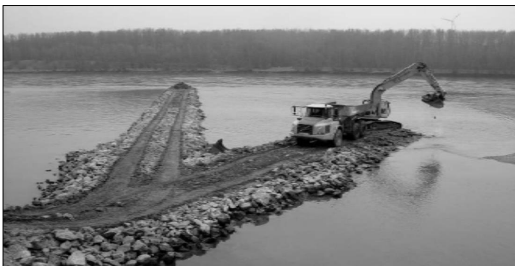
Figura 2.4-8 Constructia caii de rulare
