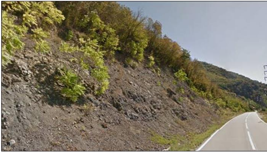
sector km 69+200 – km 69+700
