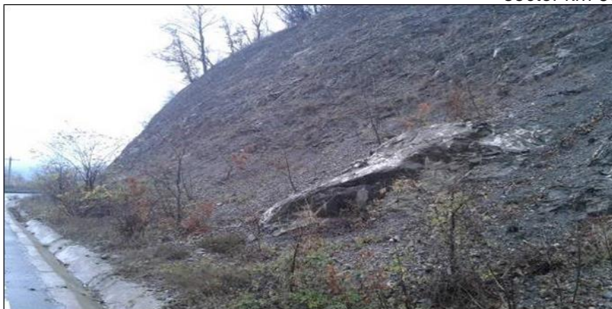
sector km 66+000 – km 66+400
