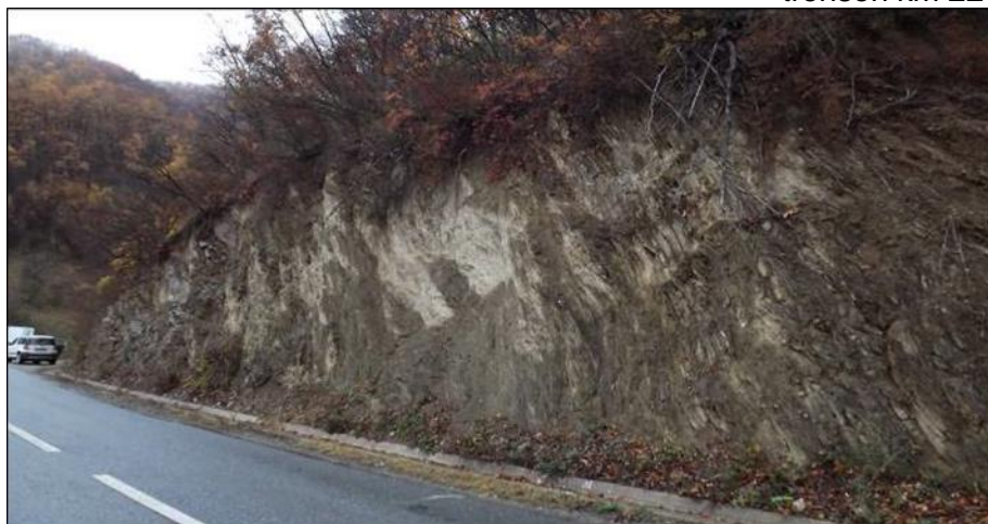
sector km 27+600 – km 28+150
