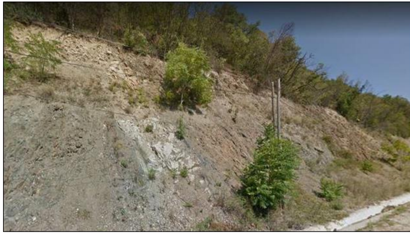
sector km 83+700 – km 84+200
