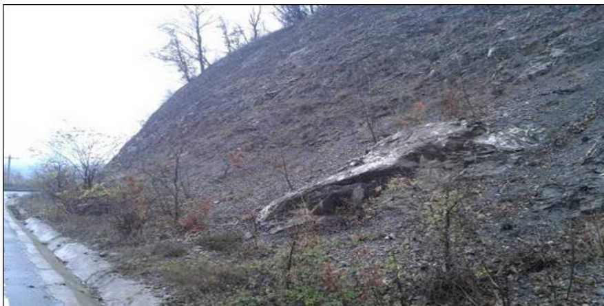
sector km 66+000 – km 66+400
