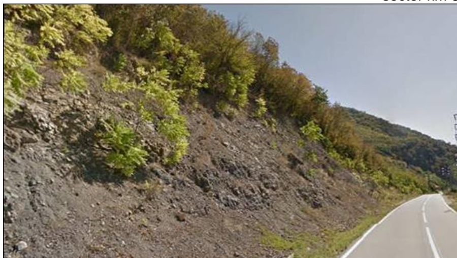
sector km 68+100 – km 68+400
