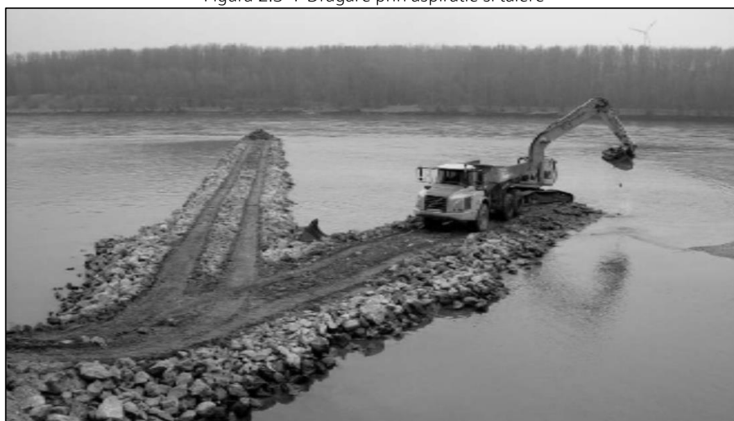
Figura 2.3-8 Constructia caii de rulare
