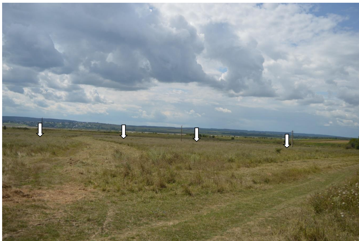
Figure 11. Baraj mal drept
