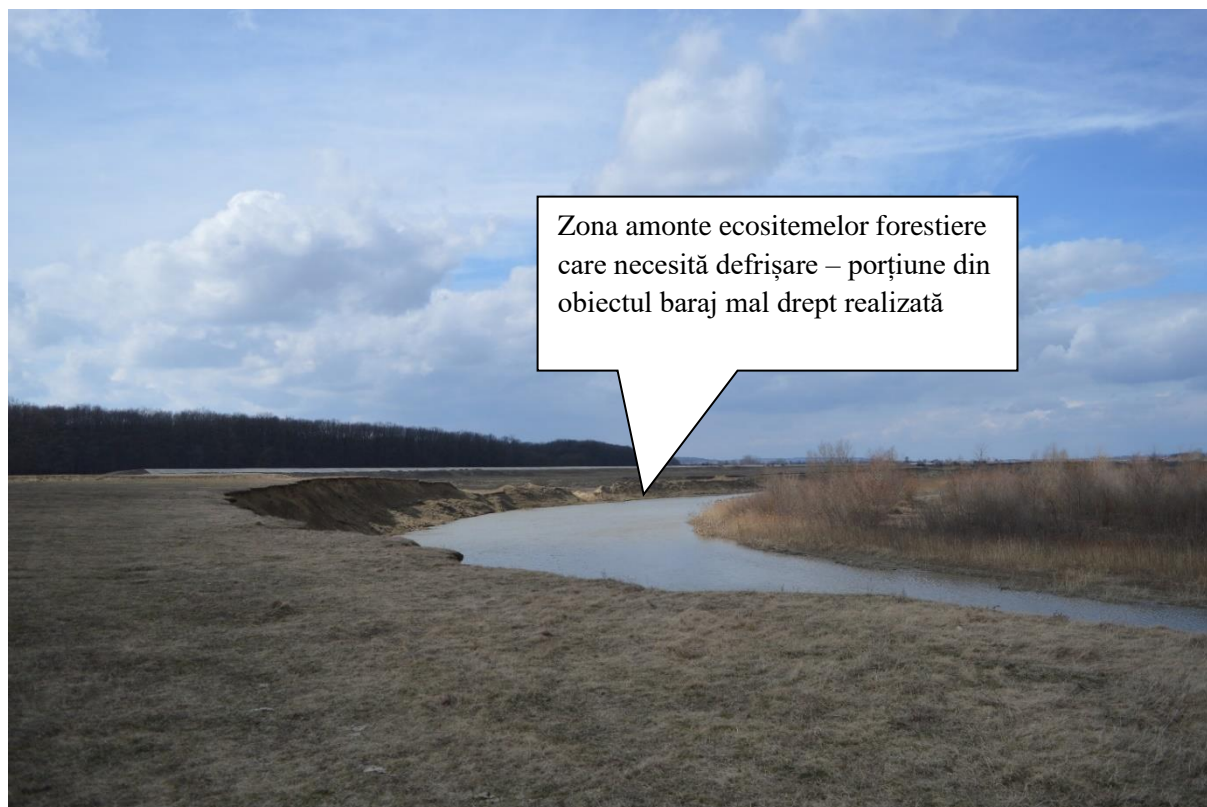
Figure 16. Baraj mal drept – zona amonte
