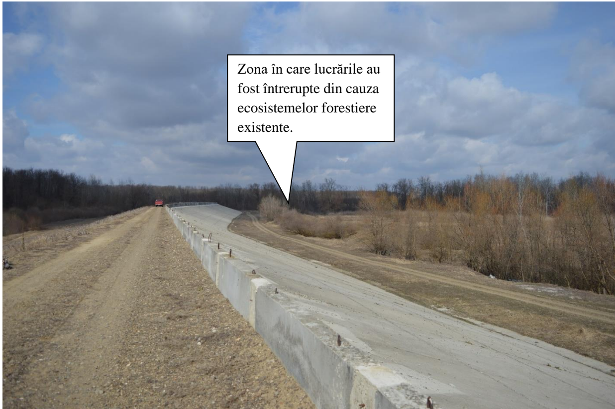
Figure 14. Baraj mal drept
