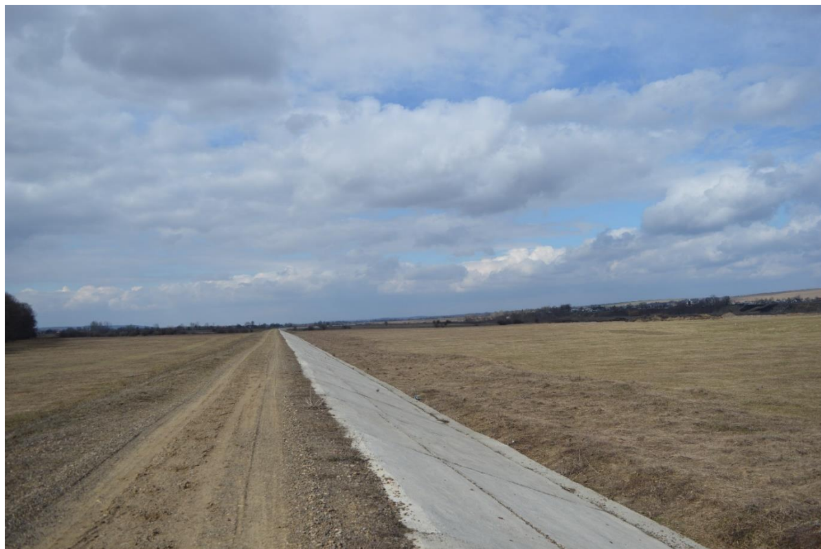
Figure 18. Baraj mal drept – zona amonte
