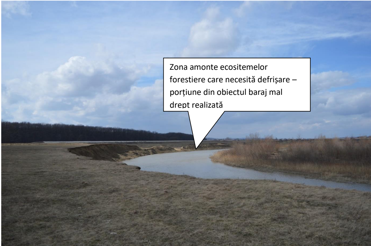
Figure 12. Baraj mal drept – zona amonte
