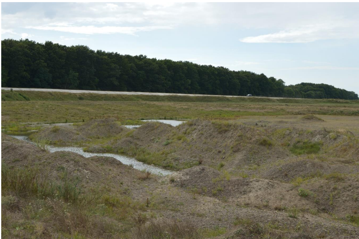
Figure 13. Baraj mal drept – zona amonte
