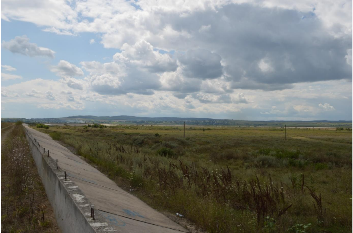
Figure 6. Baraj frontal mal stâng
