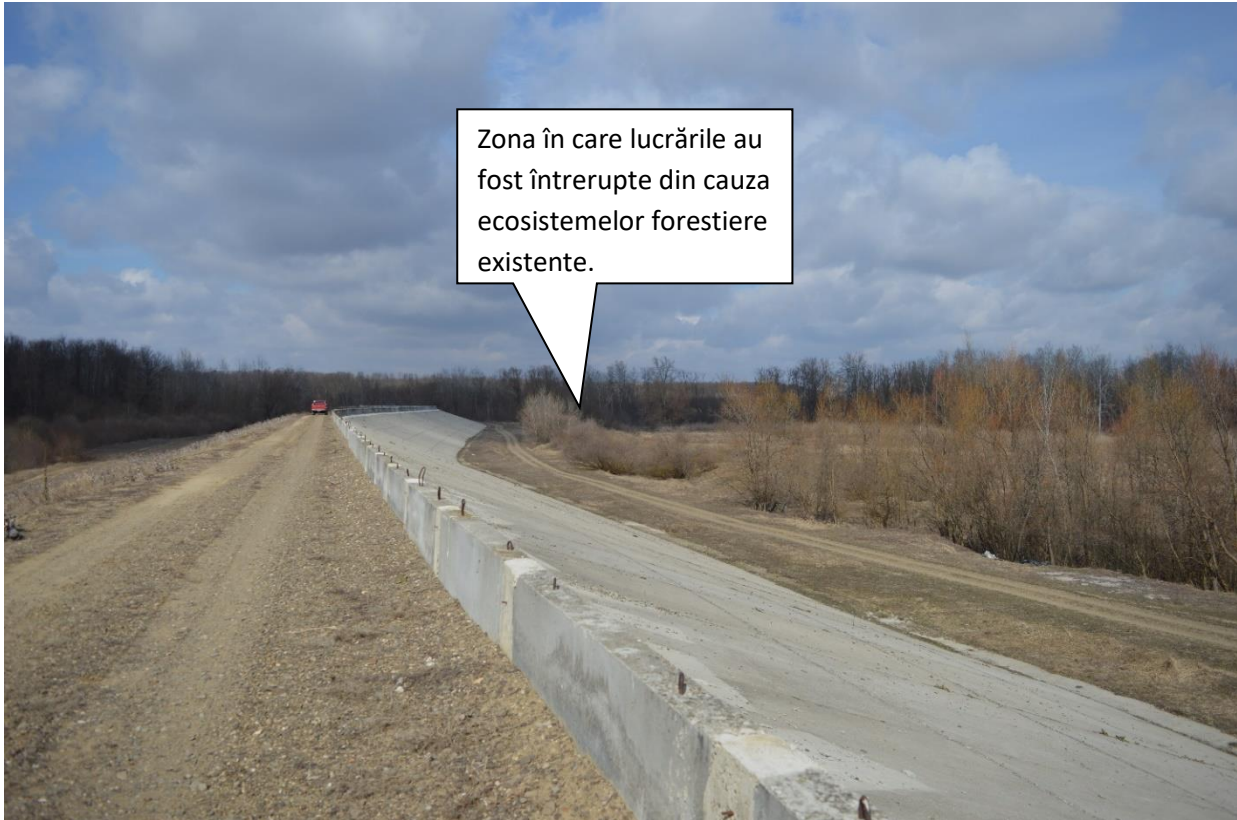
Figure 10. Baraj mal drept
