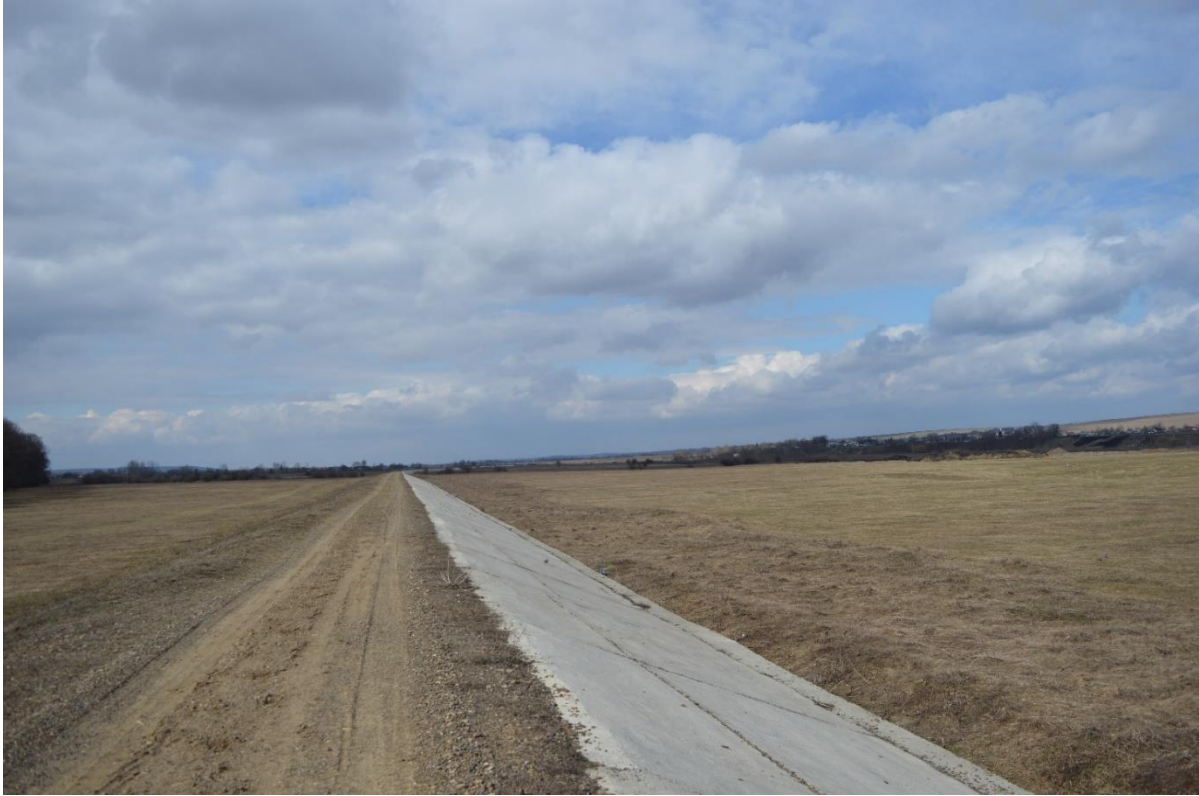
Figure 14. Baraj mal drept – zona amonte
