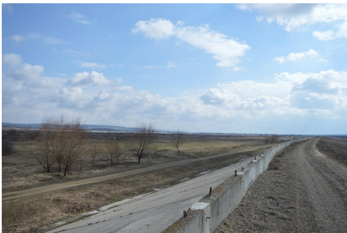
Figure 9. Baraj mal drept
