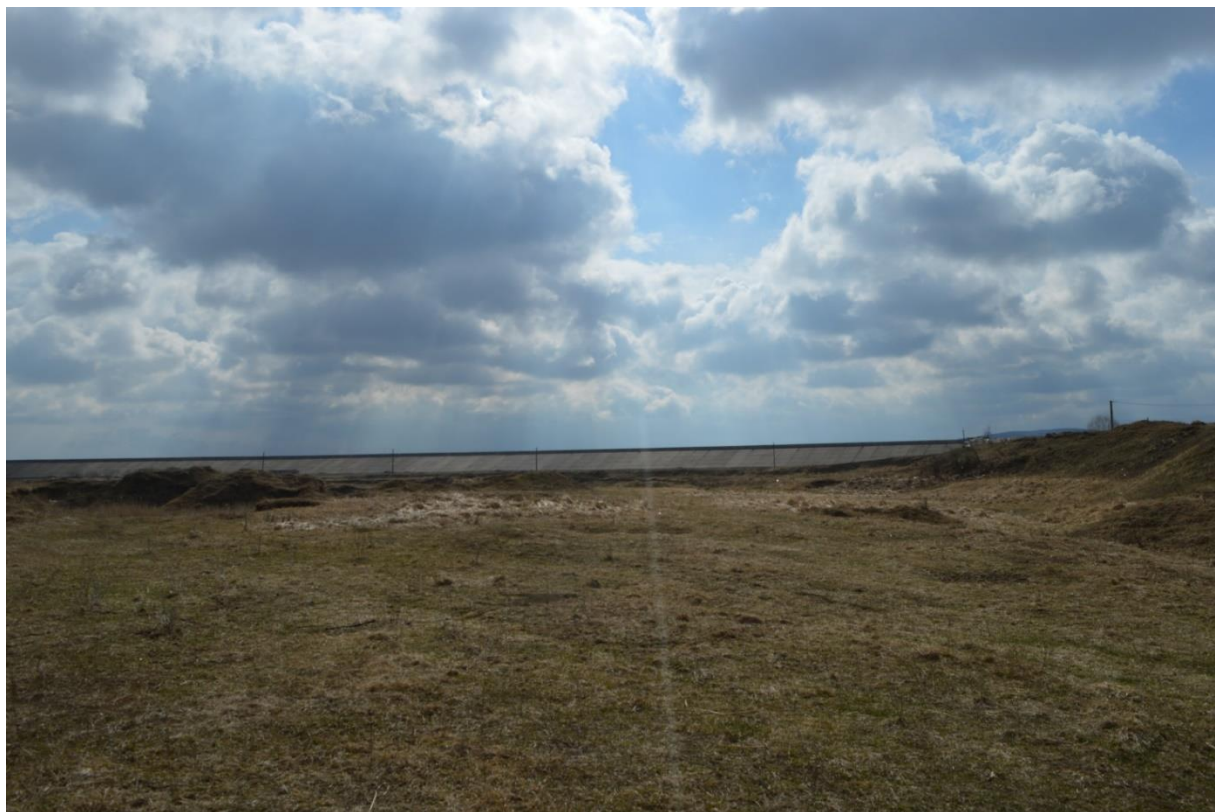
Figure 8. Baraj mal drept
