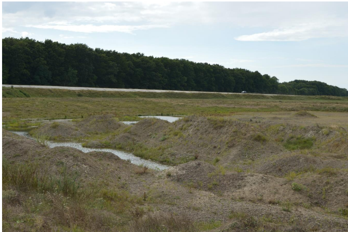
Figure 17. Baraj mal drept – zona amonte
