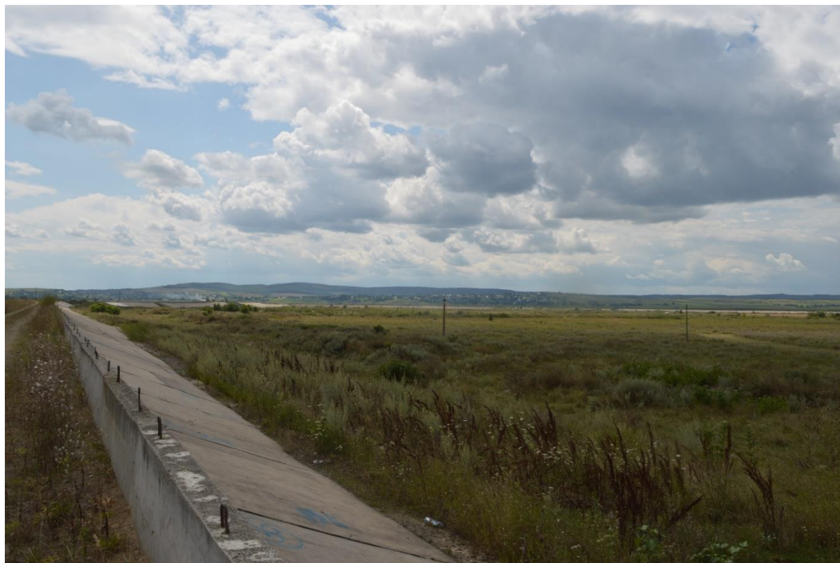
Figure 10. Baraj frontal mal stâng
