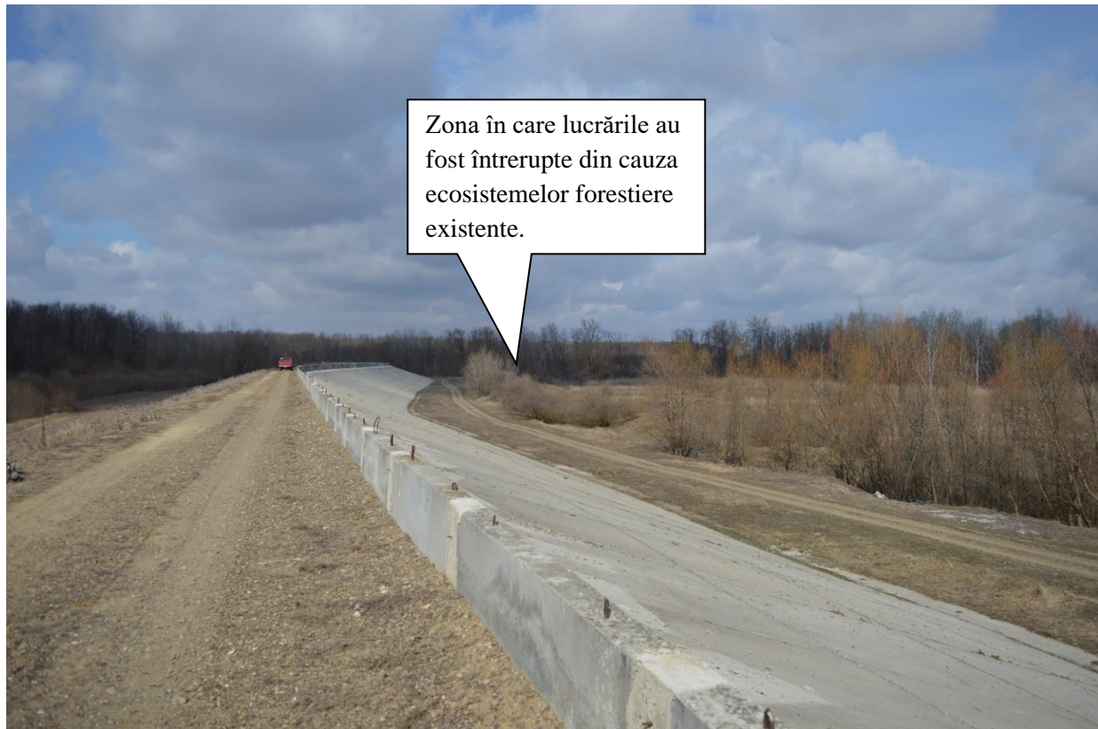
Figure 14. Baraj mal drept
