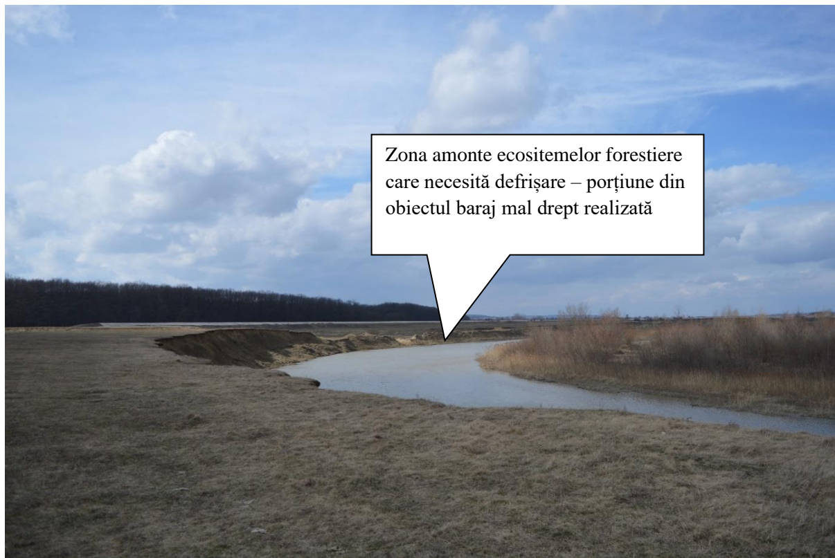
Figure 16. Baraj mal drept – zona amonte
