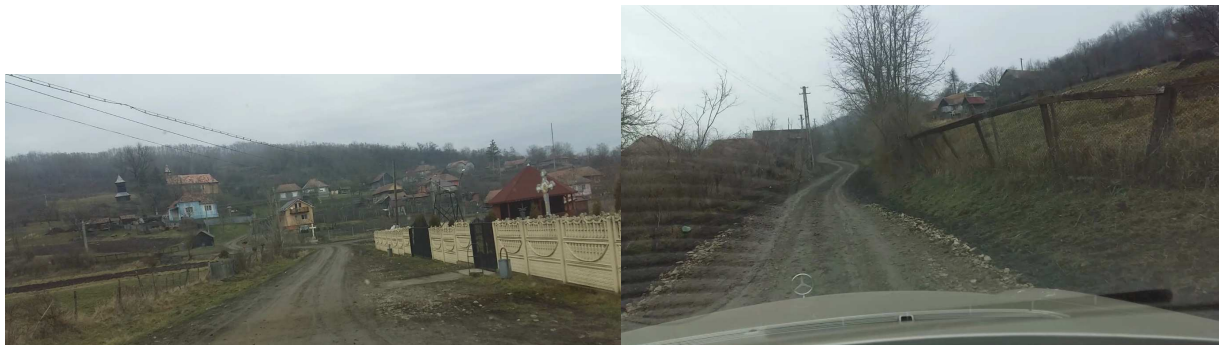
Drumuri satești degradate
