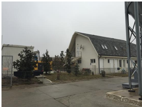
Fig.13 – Pavilion administrativ/filtru sanitar
