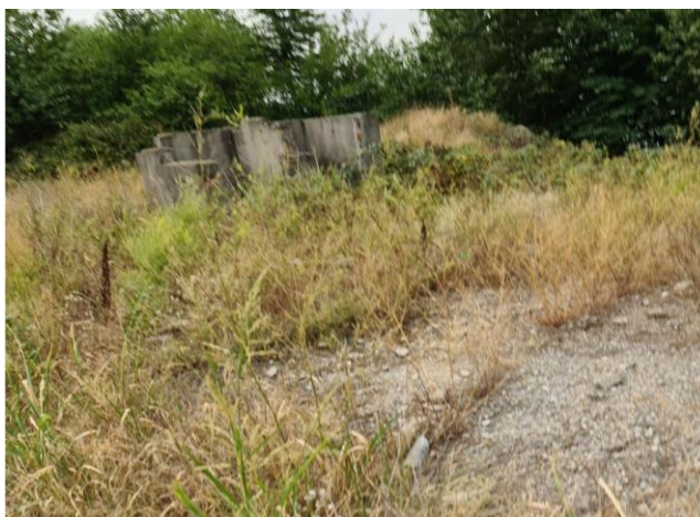
Relevu Fotografic – Constructii partial demolate
