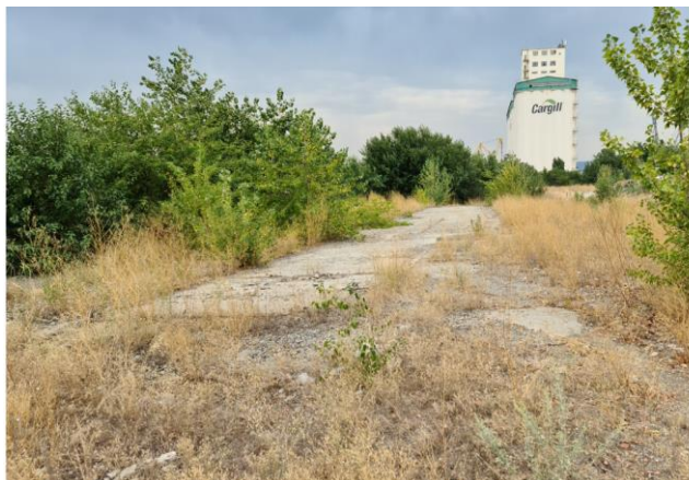
Relevu Fotografic – Platforma betonata partial demolata
