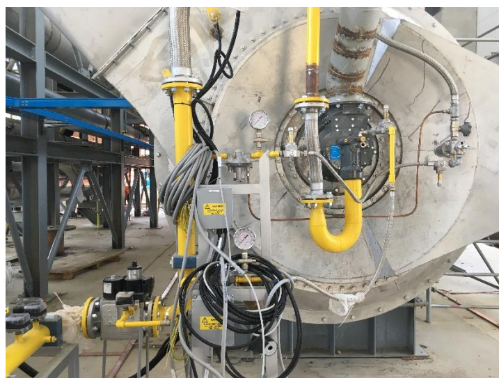
Camera de combustie/Arzator gaz metan
