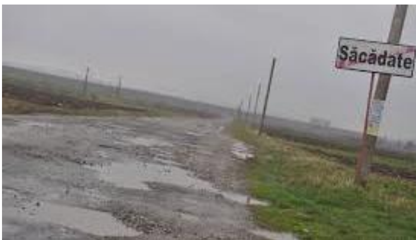
Figura 54: Amplasament Conducta de aductiune noua Bradu-Sacadate (localitatile Bradu – Sacadate, UAT Avrig, judet Sibiu)
