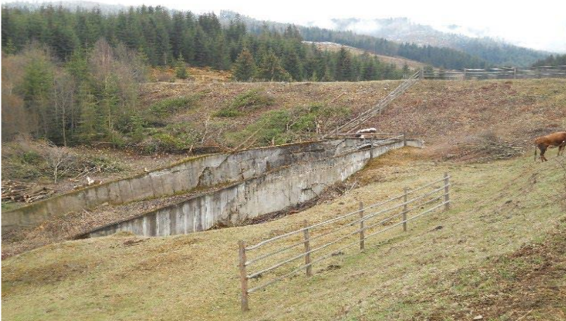
Baraj aval-parament aval
