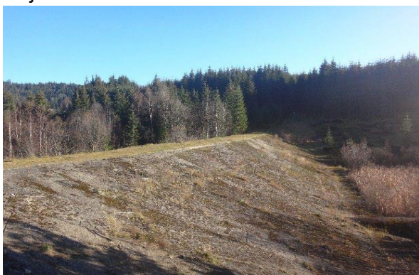
Baraj aval-parament amonte
