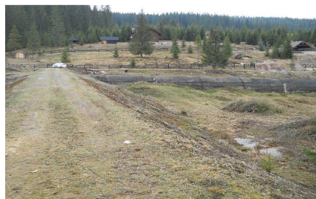
Baraj amonte -umar stang
