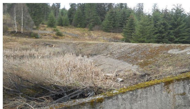
Baraj amonte-parament aval
