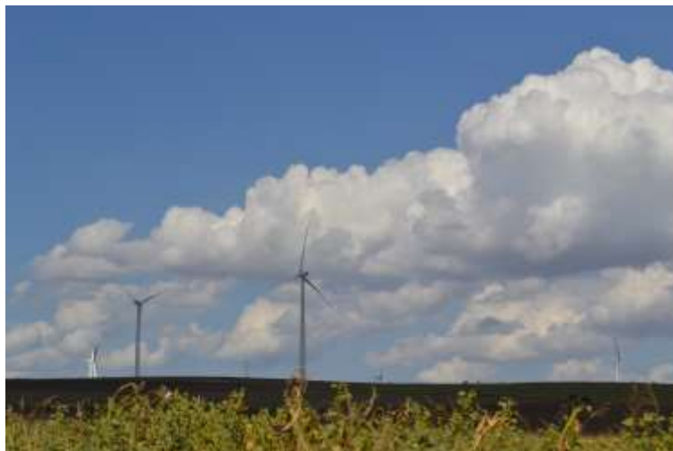
Fig. 2 – imagini parc eolian Ground Investment Corp – la finalizarea constructiei
