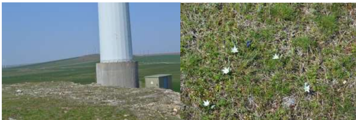
Fig. 2 -3 – platforma turbina Green Energy
