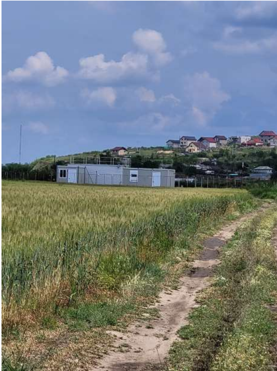
Aspect vegetatie – statia de epurare
