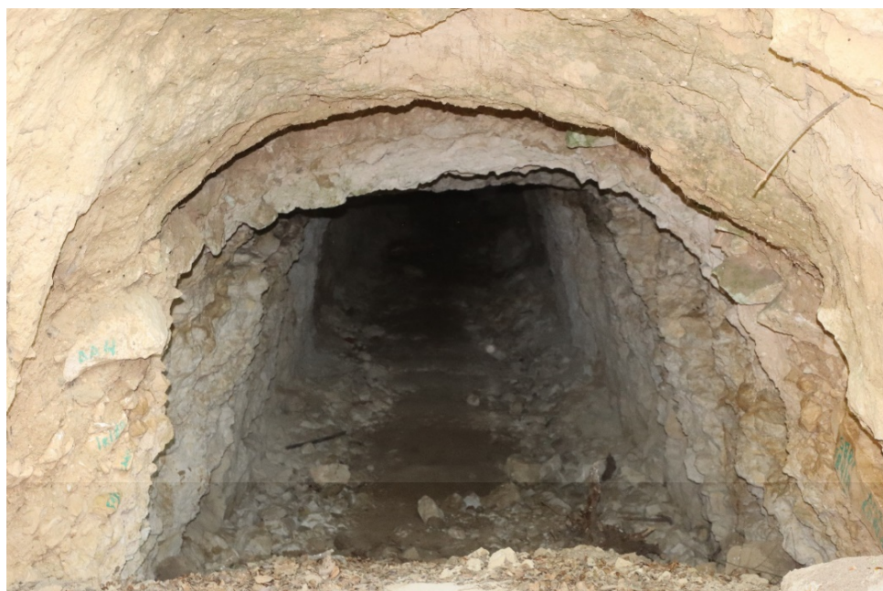
Aspect al intrarii in galeria de mina ((foto original SCBIM AON)
