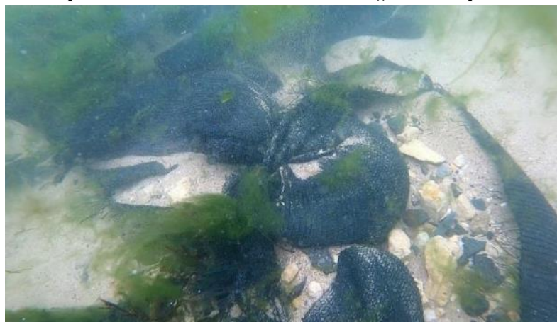
Aspect al cosurilor deteriorate
