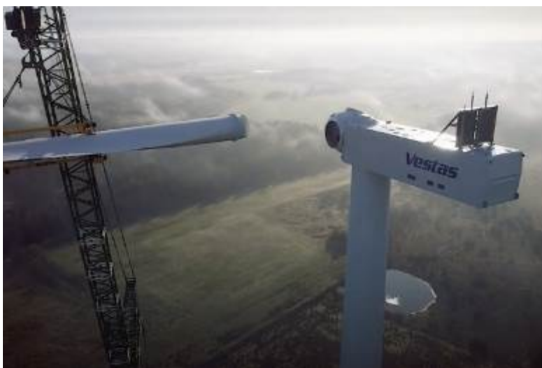
Instalare turbina (Sursa: https://www.windpowermonthly.com/ )
