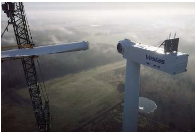
Instalare turbina Vestas V162 (Sursa: https://www.windpowermonthly.com/ )
