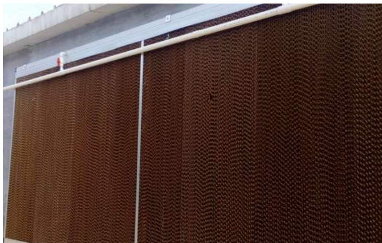
Fig.9 – panouri PAD (faguri)
