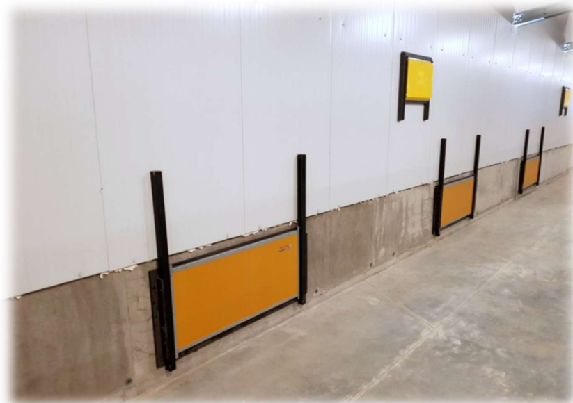
Fig.7 – Usi de acces a gainilor in padoc
