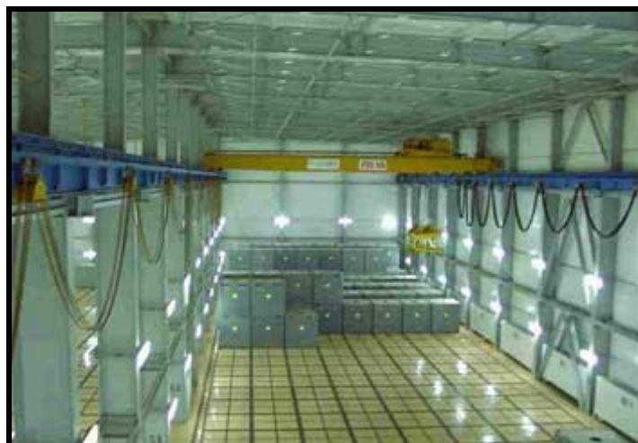
Figure 6 Temporary storage in the storage facility at Kozloduy NPP site
