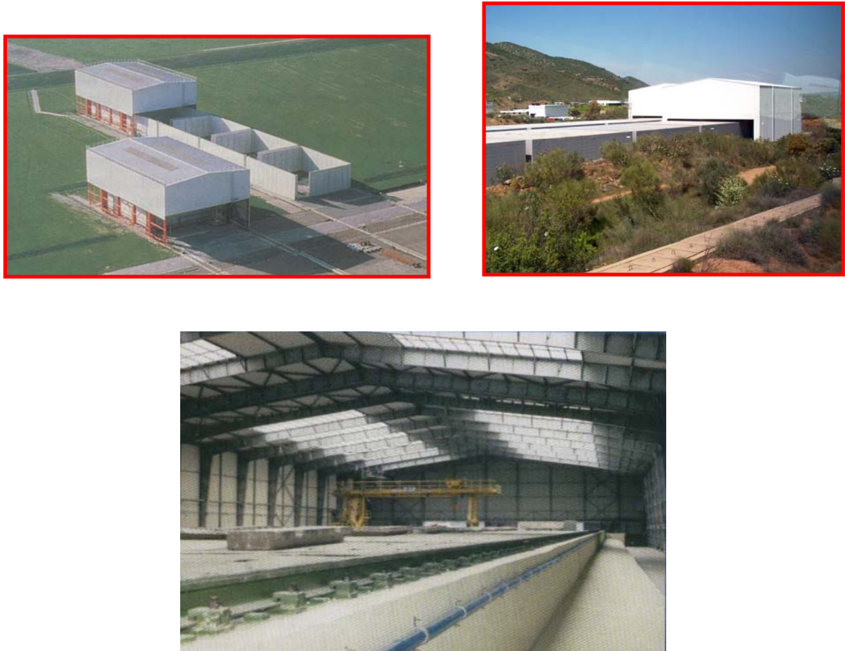
Figure 12 Modern repositories for low and intermediate RAW with protective structures during the period of operation a) Center La Obe – France, b) El Cabril – Spain, c) Mochovce – Slovakia.
