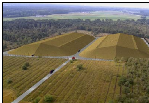
Figure 10 Sealed modular trench type repository with a built multibarrier protective cover
